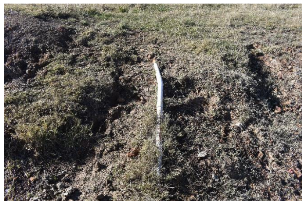
Figure 42: South Creek 3 Antenna Complex – Partially buried PVC conduit between metal shed and former location of Antenna X 3
