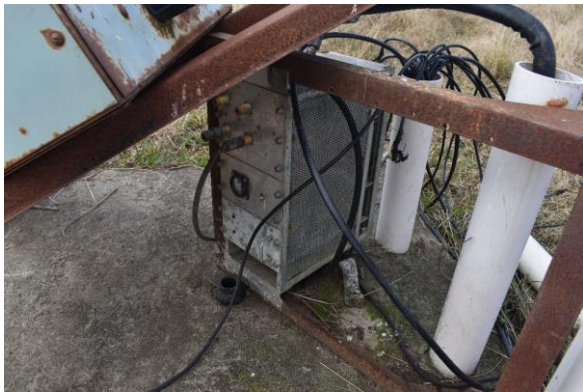
Figure 57: South Creek 4 – Detail of compressed air hoses and cut electrical connections at base of fuse box (or similar piece of equipment)
