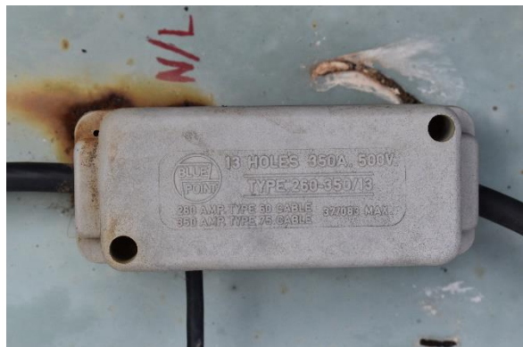
Figure 52: South Creek 4 – Detail of one of four observed neutral links
