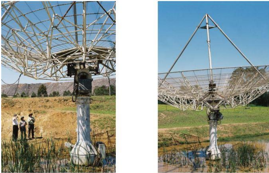
Figure 59: View of antenna X 4 in c.2004/early 2005 before removal 70
