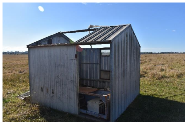
Figure 36: South Creek 3 Antenna Complex – metal shed
