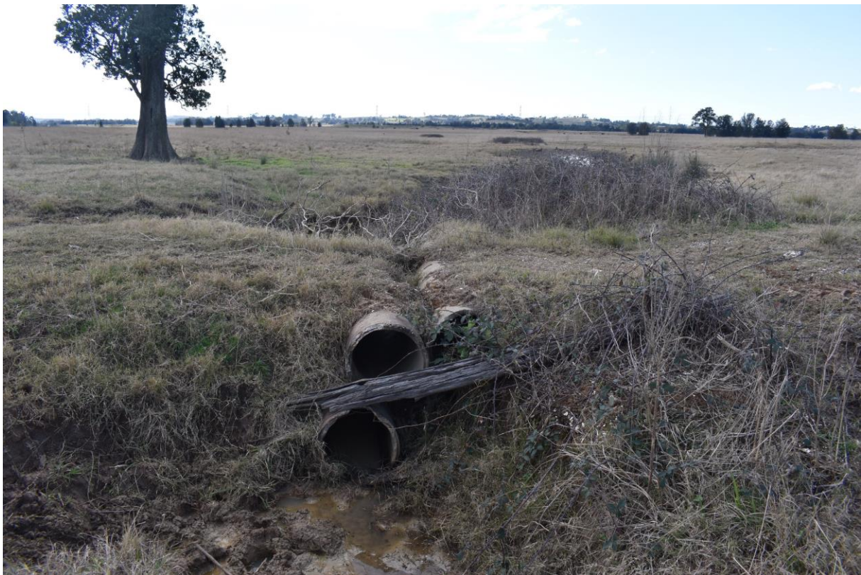
Figure 65: Former vehicle crossing over unnamed watercourse
